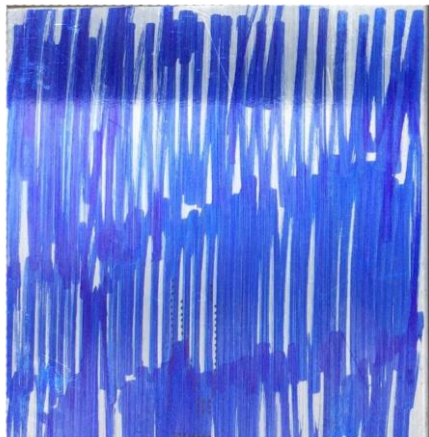
Prepped for sandblasting
